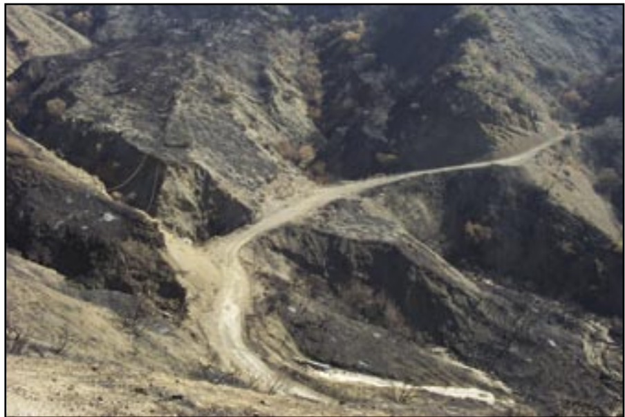
Figure 93—Removing accumulated sediment to ensure culvert capacity prior to seasonal storms can reduce the risk to the transportation infrastructure.
