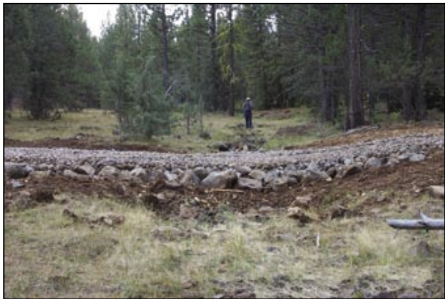
Figure 69a—Completed armored rolling dip.
