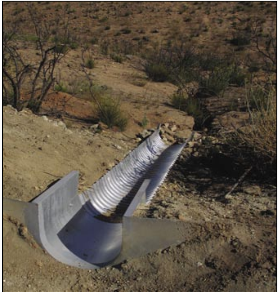
Figure 70—Metal roadside drain.
