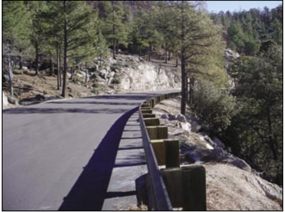
Figure 74—Imbricated rock level spreader used by FHWA in areas that burn often and control of water on the fillslope is critical.
