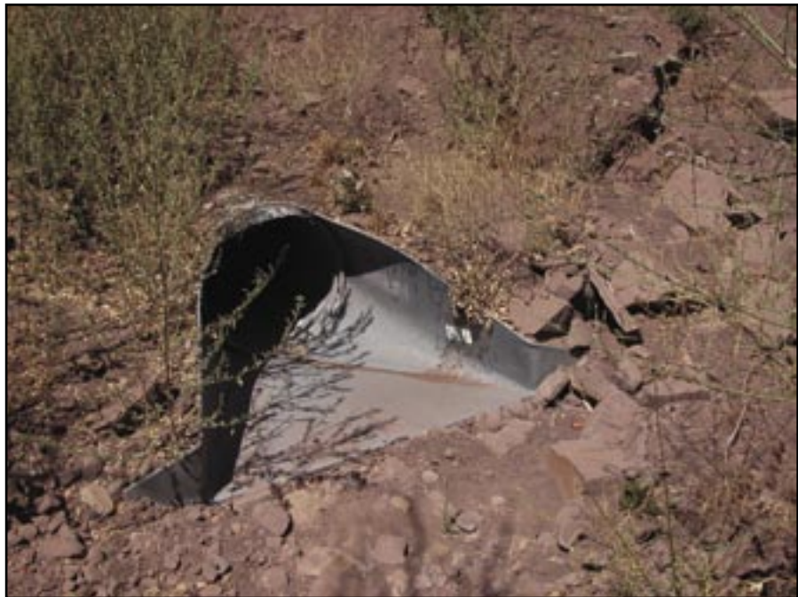
Figure 78—Metal end sections are attached to culvert inlets to improve the hydraulic efficiency and reduce the potential for plugging.
