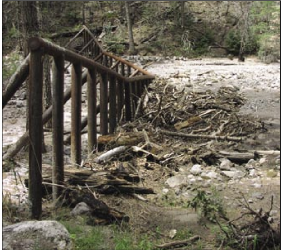
Figure 83—Debris rack effectively trapping material from plugging the culvert.
