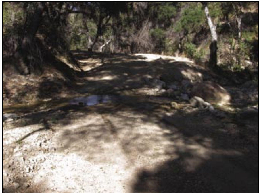
Figure 76—Low-water stream crossing replaces a 24-inch culvert.
